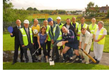
Councillor Eric Thomson cutting the turf for work to begin on the houses and sports pitch at Kirkmichael in Helensburgh.
